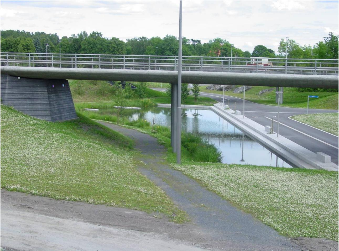
FIGURE 3. A wet pond receiving highway runoff and located in a property development, Fornebu, in Oslo, Norway. The area was until 1998 the airport of Oslo. The “permanent water volume” is in this case compared with the “storage volume” a dominating feature.
