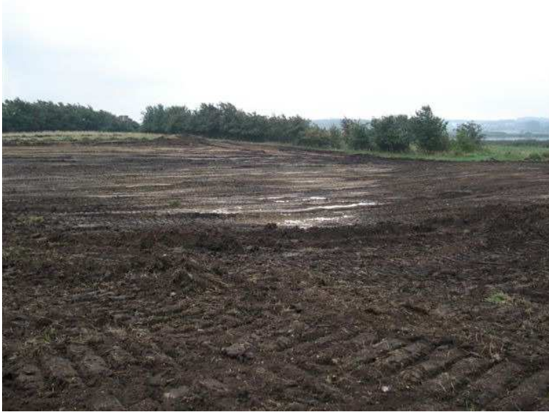
23.08.2007 – Mould removed from area
