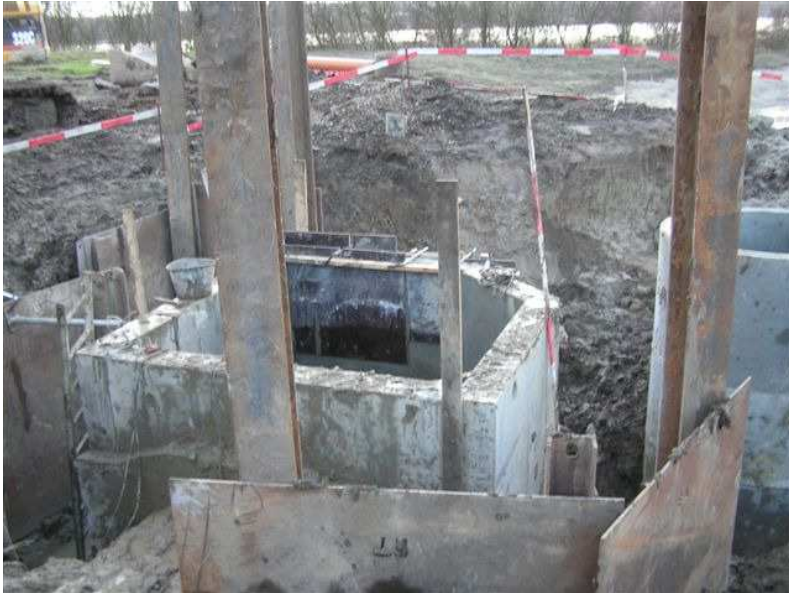
04.12.2007 – Construction of Inflow structure
