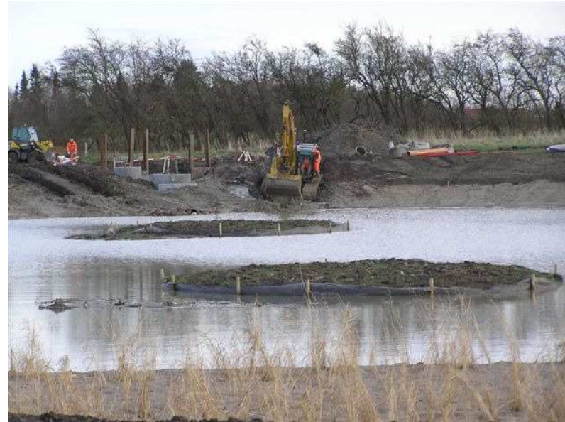
04.12.2007 - Construction of inflow structures in the background
