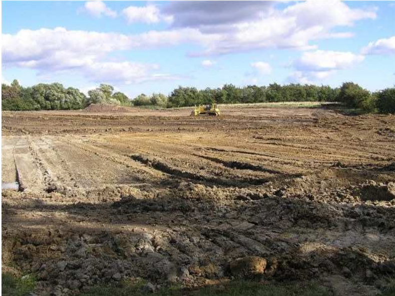
28.08.2007 – Surface modelling of pond bottom
