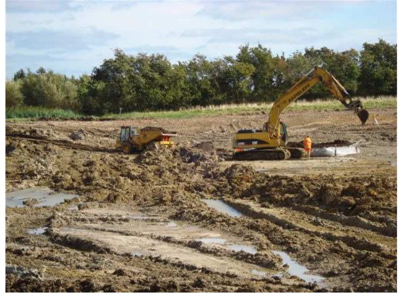
12.09.2007 – Construction of polder
