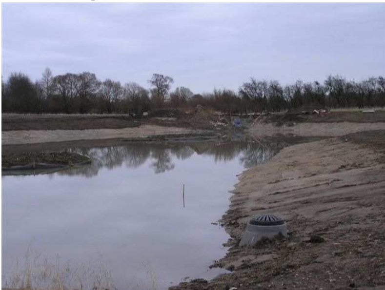
30.10.2007 – Outflow grating for optional filter by-pass in the foreground
