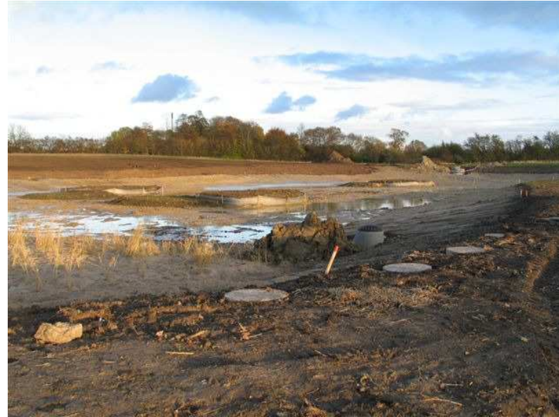
30.10.2007 - Drainpipe cleaning access in the foreground
