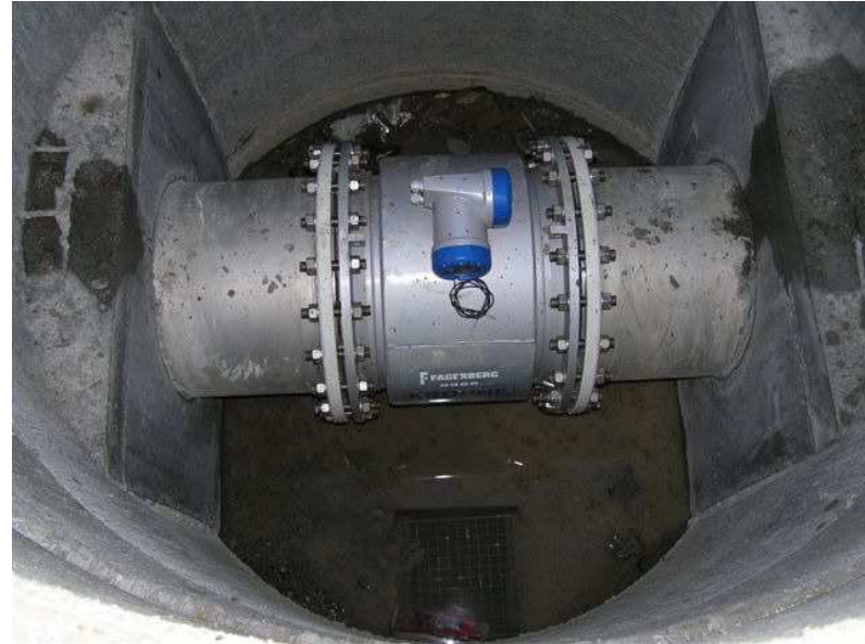
04.12.2007 – Flow meter in Inflow structure
