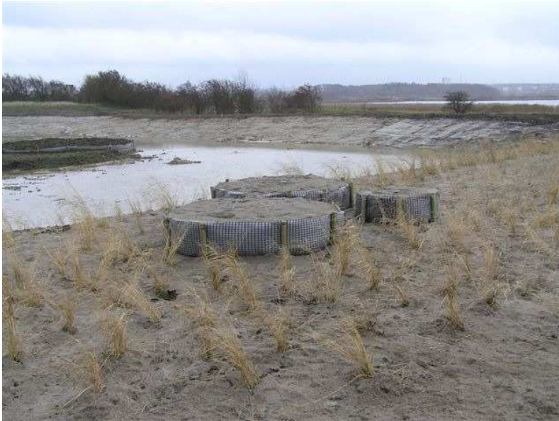
08.11.2007 – Vertical filters and horizontal filter planted with reed
