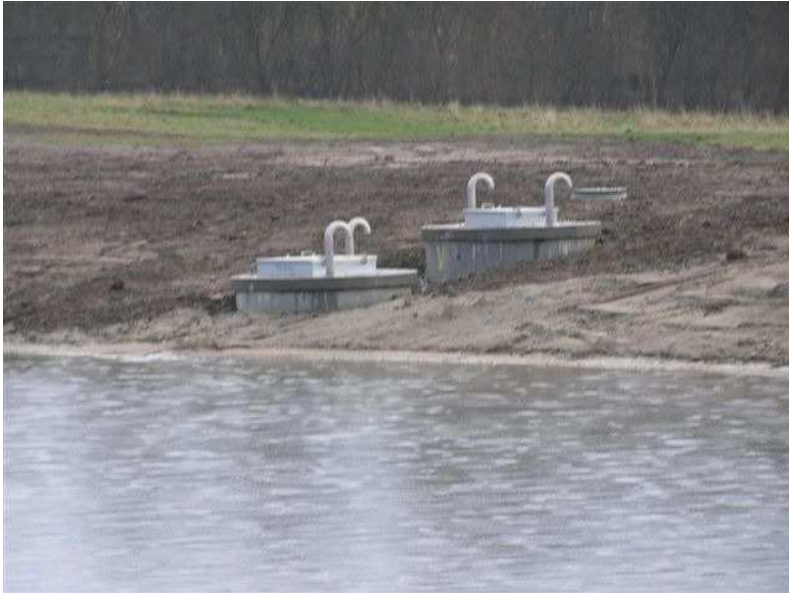
15.01.2008 – Valve- and flow meter structure (Inflow structure)
