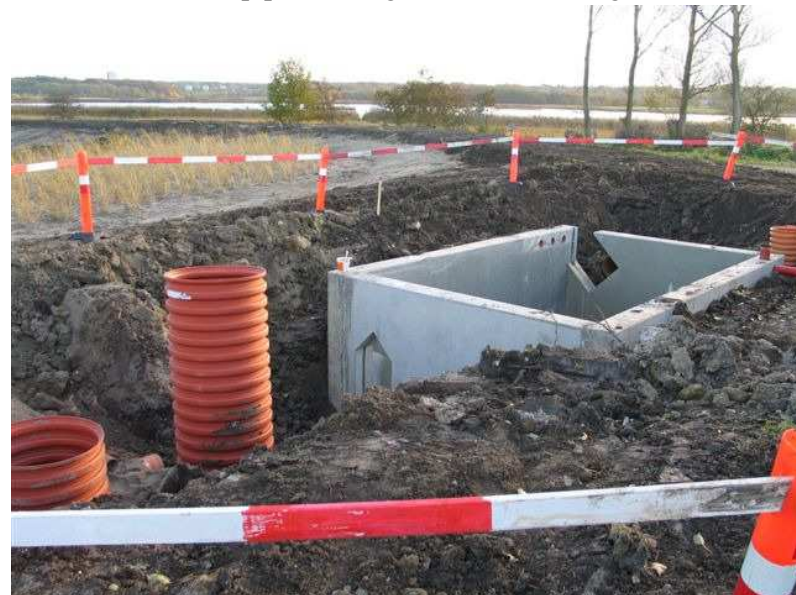
30.10.2007 – Construction of outflow structure
