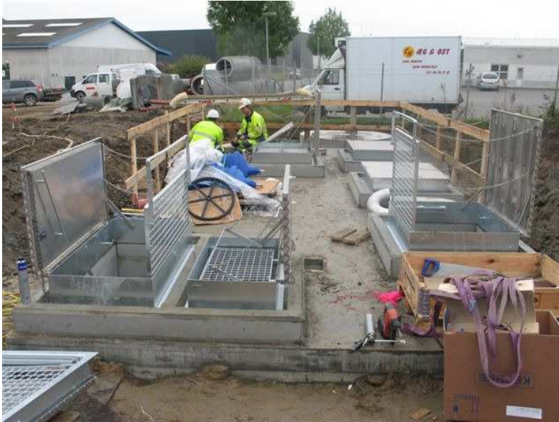
11.10.2007 – Inflow structure near completion
