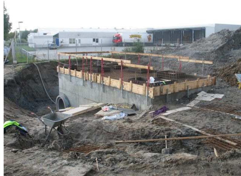
29.09.2007 – Construction of inflow structure
