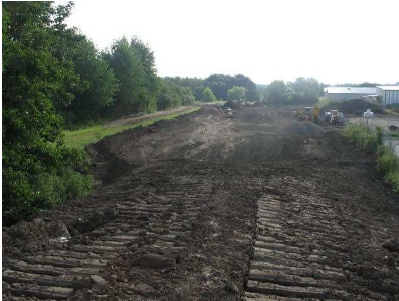
08.08.2007 – Mould removed from area
