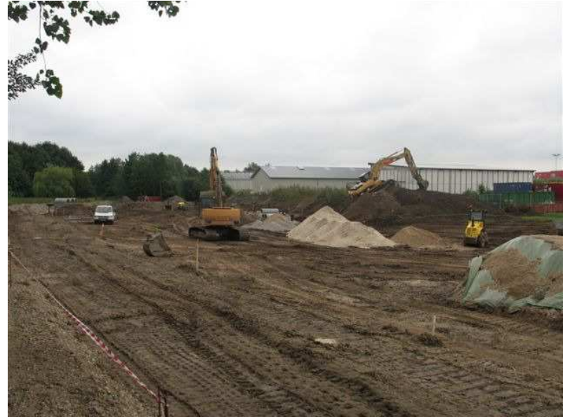
21.08.2007 – Earthwork in progress
