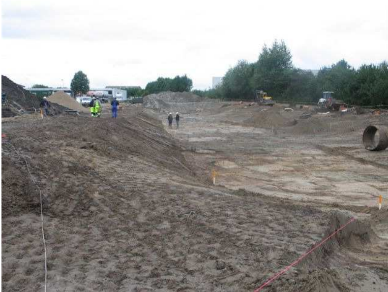
11.09.2007 – Excavated to Pond bottom level
