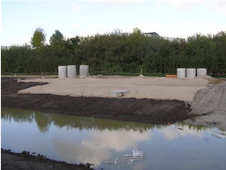
06.10.2007 – Sand filters constructed
