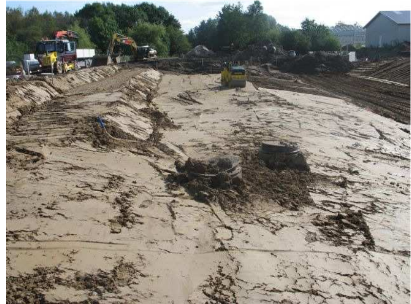
13.09.2007 Construction of clay membrane
