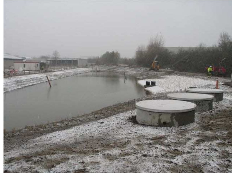
14.11.2007 – Structures for handling outlets from various sections
