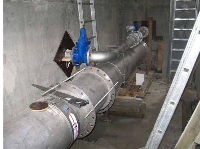
11.10.2007 – Inflow structure, stainless steel pipe installation
