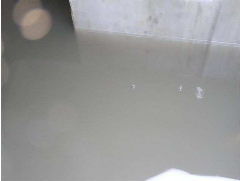
26.02.2008 – Testing inflow structure tightness
