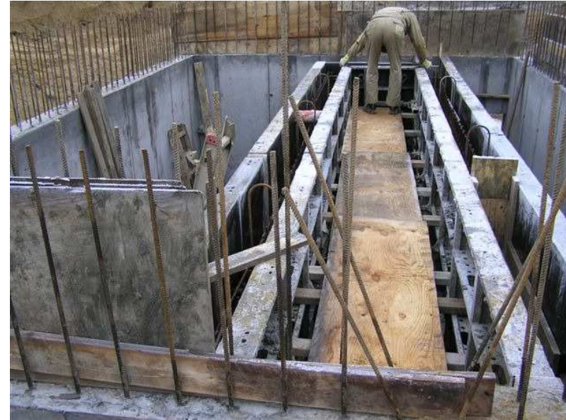
19.12.2008 – Construction of inflow structure
