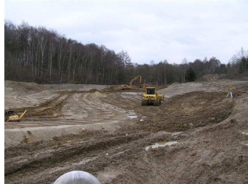
11.03.2008 – Construction of clay membrane (more drain installed)
