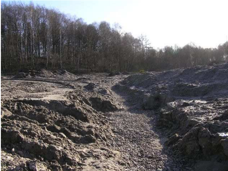
07.02.2008 – Draining system installed under pond bottom
