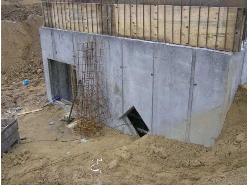
19.12.2007 – Construction of inflow structure
